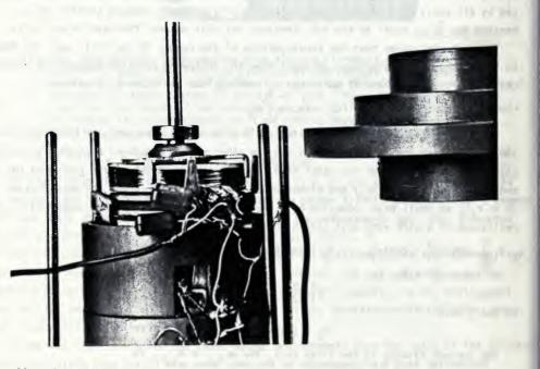
Fig. 14. - One of the Bosch generators (the tenth in VENETIN COLIU - I) with the original Bosch coil on which additional windings were wound. coils by coils wound without holders. The new nine coils had about 3000 windings each of wire of diameter 0.22 mm, resistance about 400  $\Omega$  and inductance about 1 H.
