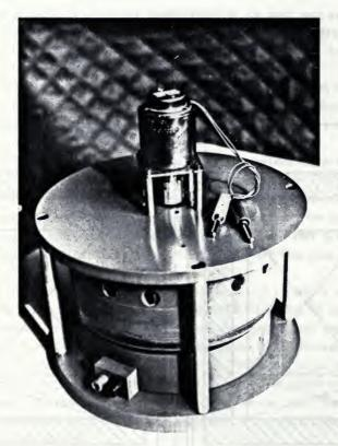
Fig. 18. - The second VENETIN COLIU machine constructed by Marinov in February 1991. The d.c. motor on the top drives the rotor.
